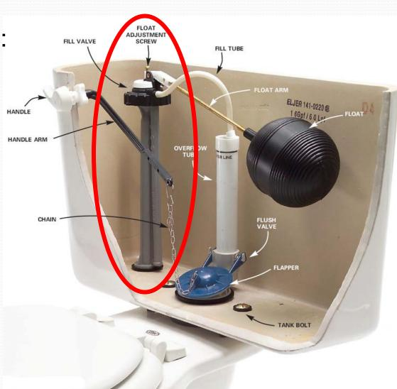
Turn off the water supply, flush the toilet, and sponge the remaining water from the tank.
