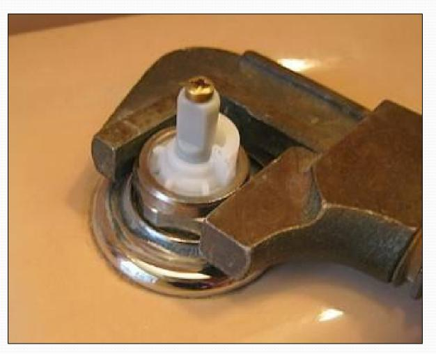
Loosen retaining ring and remove.
