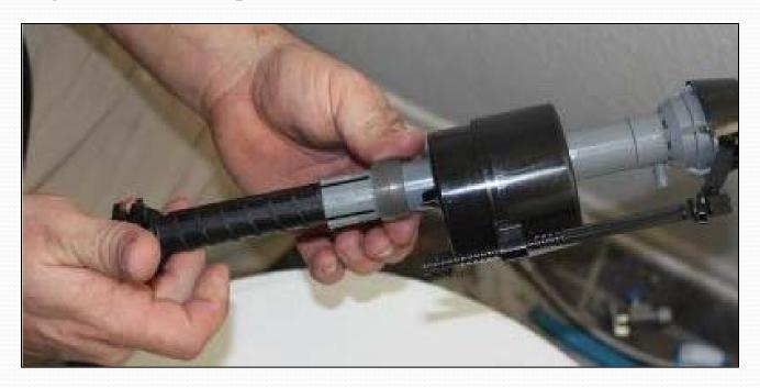
Prepare the new fill valve by adjusting the height of the fill valve as necessary.
