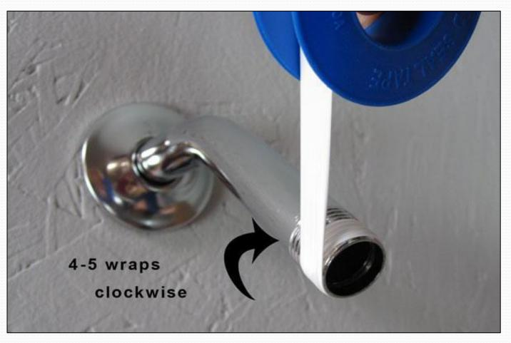
Wrap Teflon tape around shower arm threads 4 - 5 times in a clockwise direction.
